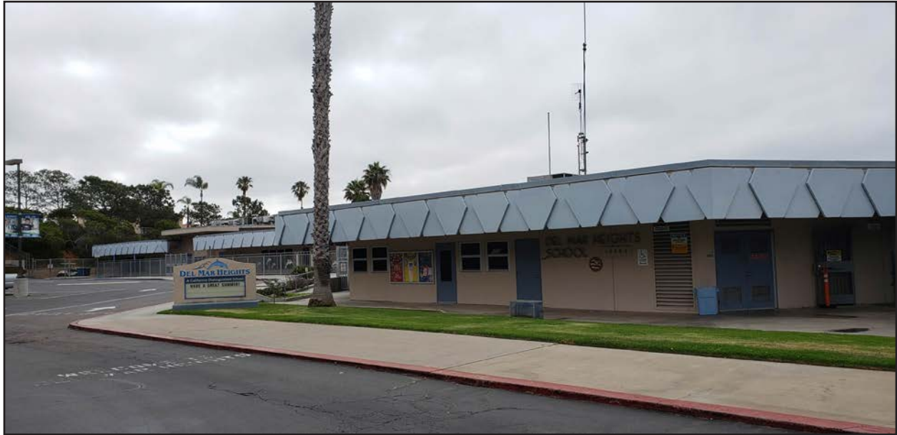
Figure 4b - Site Photographs 1. Introduction
